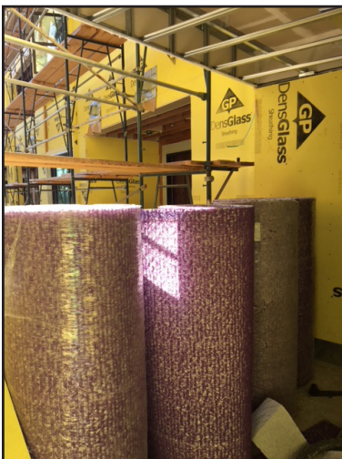
Rolls of SCM-400 staged before install
