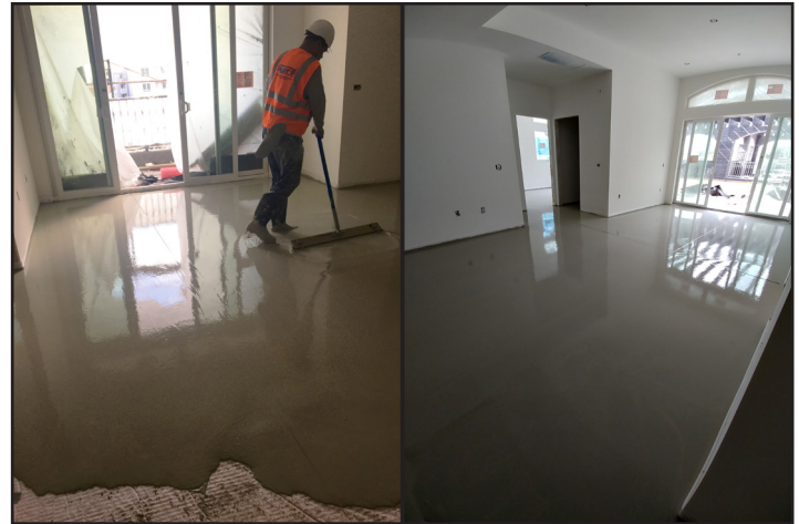
Troweling the 2010+ as it's pumped over the SCM-400
