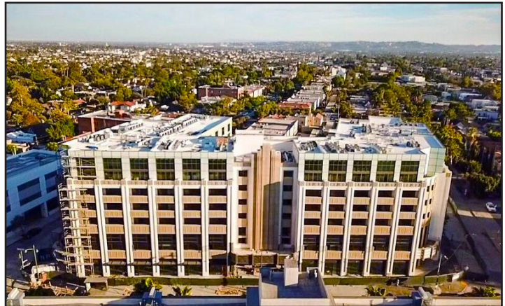
The Mansfield during construction, set in its West Los Angeles neighborhood
