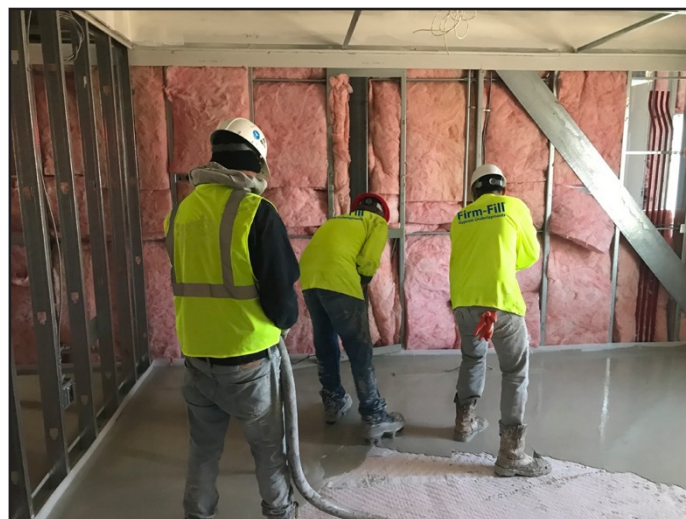
The second lift of Firm-Fill® CMD is installed over Firm-Fill® SCM-250 at 1-1/4" in depth
