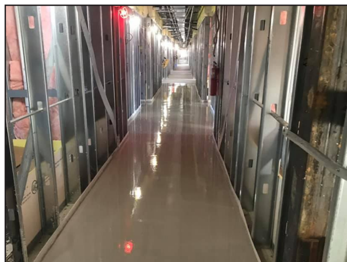
Finished pour of Firm-Fill® CMD in hallway - the gypsum dried enough to walk on within 90 minutes
