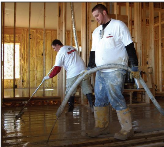
In the search for a product that would provide warm, comfortable floors and uniform heat, General Contractor Addco Builders selected **GYP-SPAN® Radiant** gypsum concrete floor underlayment. Known for its inherent high strength and energy efficiency, **GYP-SPAN® Radiant** provided a radiant heat system that ensured even heat transfer in every room.
