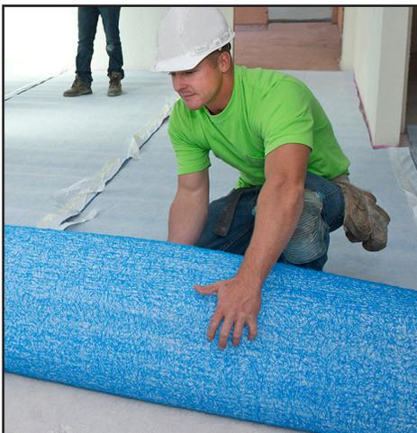
To Assist Quality Control, Firm-Fill® SCM-125 is Color-Coded Blue for Easy Identification
